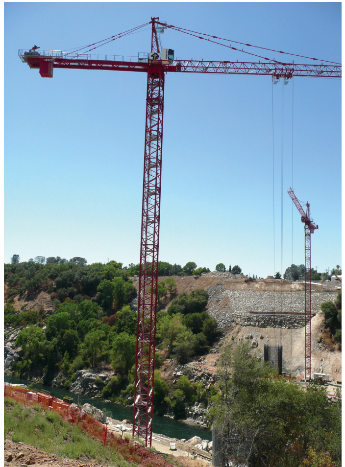
Tower cranes dwarf the bridge site, including the steel going up for the west column. Behind operator Dennis Dorton are the crane he just climbed down, steel cages for the columns and the forms for concrete the crane will lift into place.
